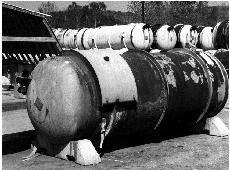
A depleted uranium hexafluoride (DUF 6 ) storage cylinder with external corrosion (rust) and a patch used to repair a breach, Portsmouth Gaseous Diffusion Plant, Portsmouth, Ohio. More than 16,000 DUF 6 cylinders (approx. 195,000 metric tons) are currently stored at the Portsmouth plant. An additional 36,000 cylinders are stored at the Paducah Gaseous Diffusion Plant in Paducah, Kentucky, and nearly 5,000 more at the Oak Ridge site in Oak Ridge, Tennessee.
