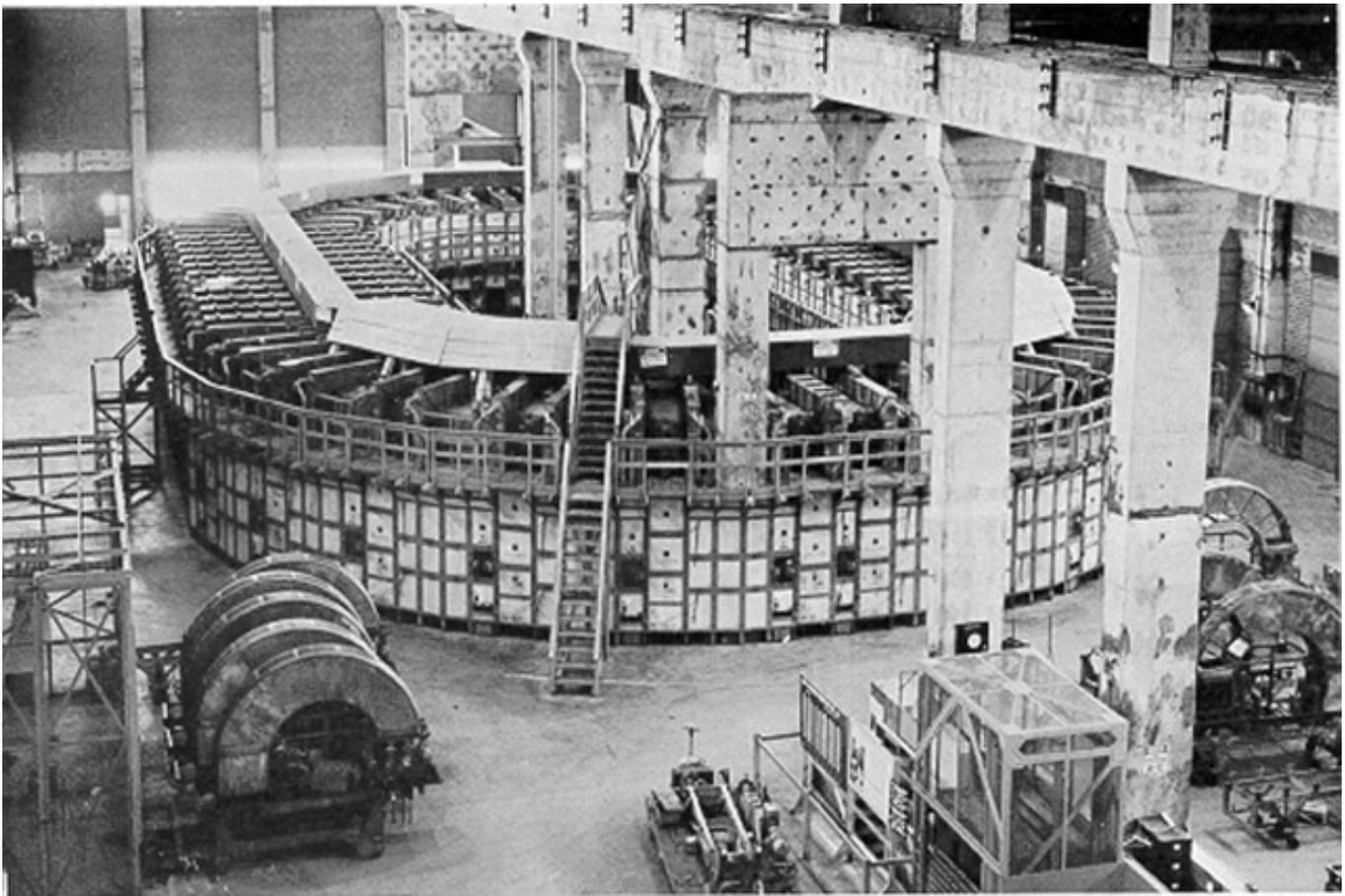
*Figure 6: The electromagnetic separations plant built at Oak Ridge, Tennessee during the Manhattan Project. These devices, also referred to as calutrons, were used in enriching a part of the uranium for the bomb that was dropped by the United States on Hiroshima. (photo taken from the website of The Manhattan Project Heritage Preservation Association online at <http://www.childrenofthemanhattanproject.org/OR/Photo-Pages/ORP-149.htm>)*
