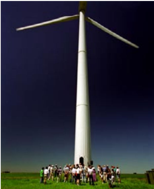
People at the base of a modern wind machine in northwestern Iowa.
