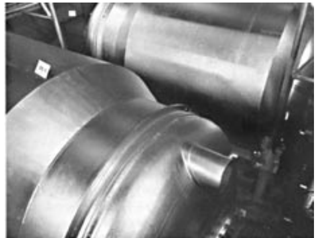
Figure 3: A close up picture of the outside of two of the diffuser stages used at the Oak Ridge uranium enrichment plant.
