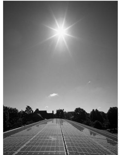
Photovoltaic panels at Oberlin College, Oberlin, Ohio. This building includes 4,682 square feet of PV panels, closed-loop geothermal wells for heating and cooling, and a wastewater treatment system modeled on natural wetland ecosystems.
