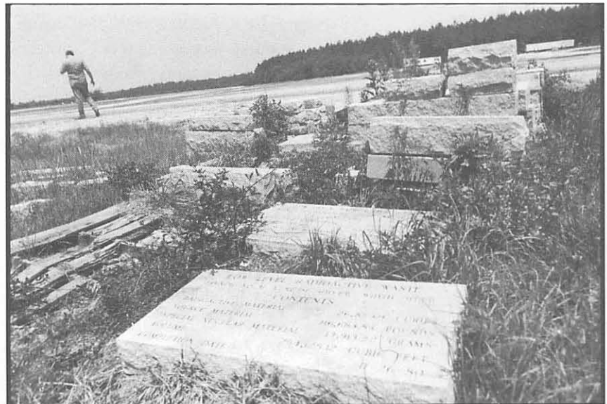
Low-level radioactive waste burial markers in Barnwell, S.C. Each headstone marks a large trench containing commercial, industrial and medical radioactive waste.
