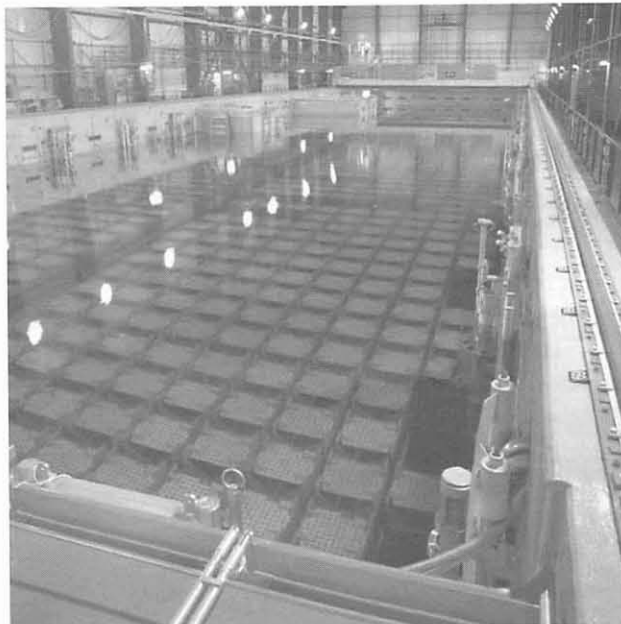
Spent fuel storage pool, COGEMA-La Hague reprocessing plant, France. Irradiated fuel assemblies are placed in baskets and stored underwater for at least two years before they are reprocessed.
