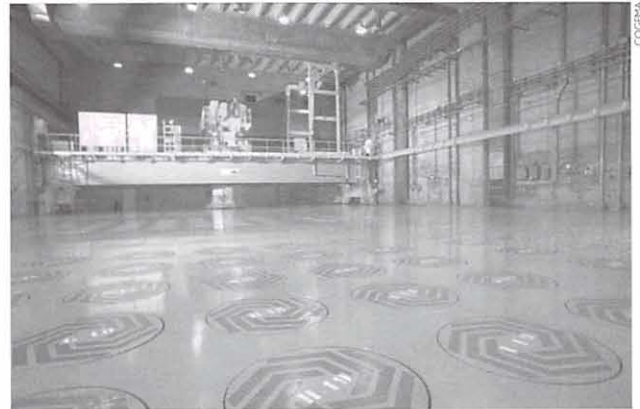
Vitrification facility storage hall, COGEMA La Hague reprocessing plant, France. This building stores highly radioactive waste, generated from the reprocessing of spent nuclear fuel, after it is vitrified and packaged in stainless steel canisters. The waste canisters are not visible in the photograph because they are stored under the floor in air-cooled dry wells.
