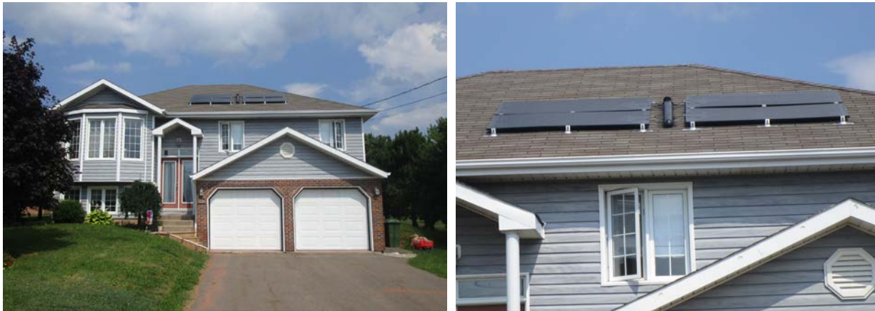
Figure III-4. Two views of solar thermal panels associated with a SunPump heat pump on Prince Edward Island, Canada. Source: SunPump Gaudin 2016 (Solar Source Ltd, PEI, Canada. www.sunpump.solar )
